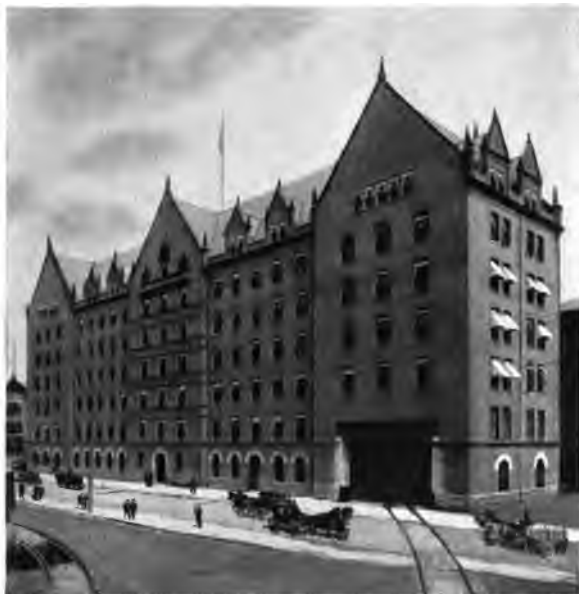
Main Office Building, Westinghouse Electric & Mfg. Co.
